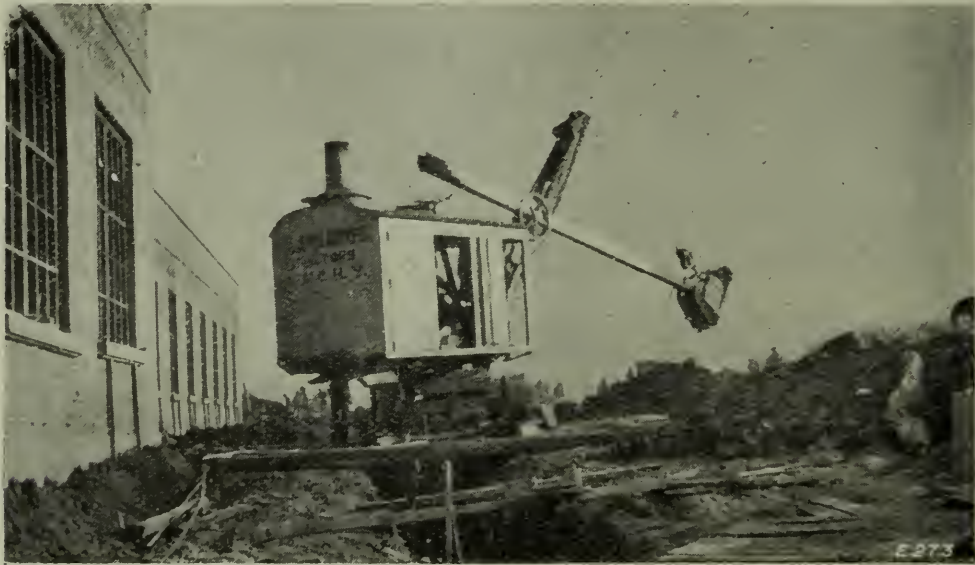
FIG. 13. STEAM SHOVEL EXCAVATING DRAINAGE TRENCH.
